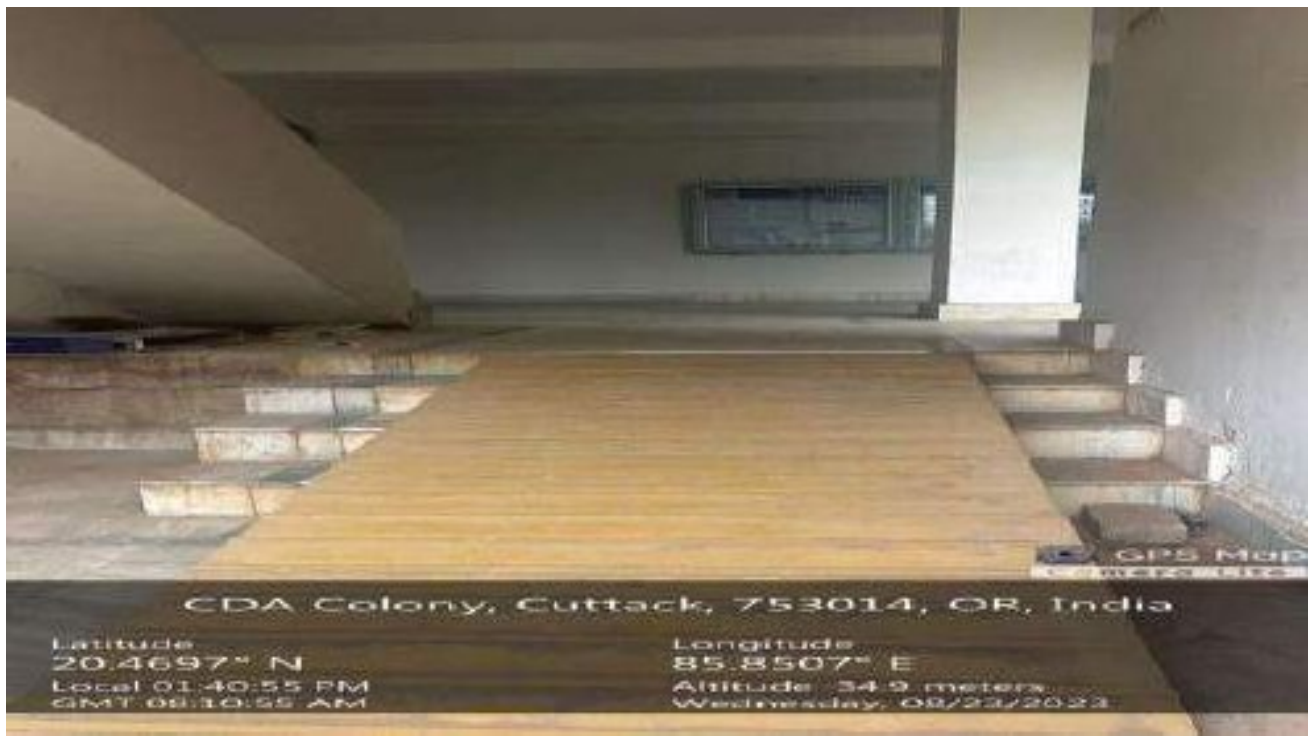
Ladder @ ABIT Main Block
