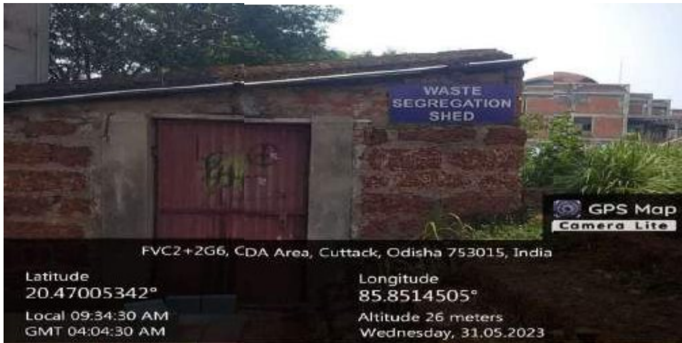
Waste Segregation Shed
