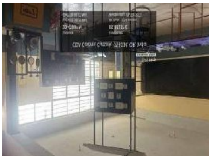
Room No E-103 Energy Conversion Device Lab
