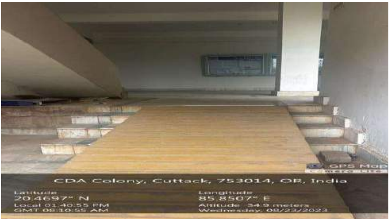
Ladder @ ABIT Main Block
